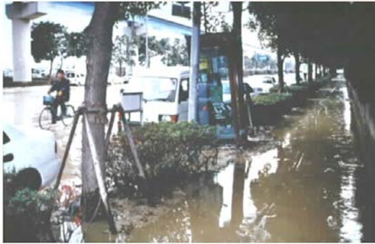
The 1995 Great Hanshin-Awaji Earthquake: Central part of Port Island, Kobe City
