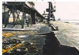
No measures have been adopted (3-A quay wall)
